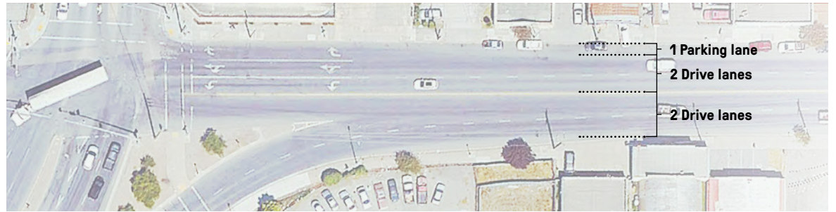
FIGURE 4.9 EAST MARKET STREET AND SHERWOOD DRIVE INTERSECTION - EXISTING CONDITIONS
