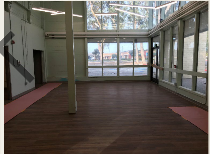
Sherwood Recreation Center Rehabilitation
