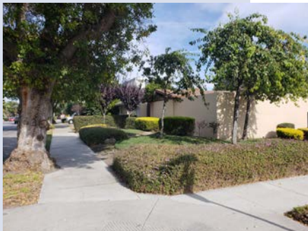
Example of a water well facility designed to be compatible with surrounding development.
