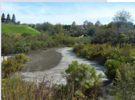
Example of supplemental stormwater detention and retention basins landscaped to have a natural vegetated appearance.
