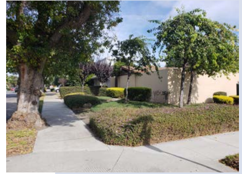
Example water well facility designed to blend with surrounding neighborhood.
