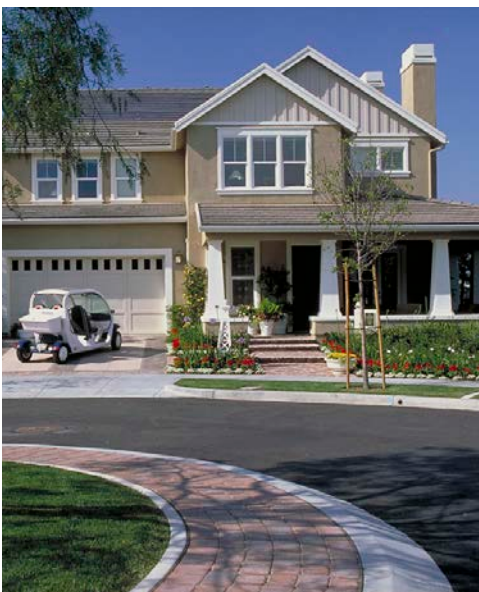
Design standards are essential to achieving the desired aesthetic envisioned for the West Area Specific Plan.
