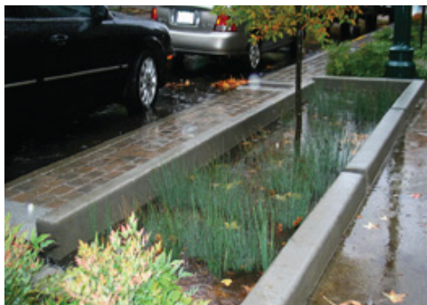
Street Infiltration Planter
