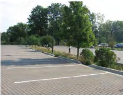
Pervious Pavement Construction
