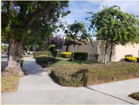
Example of a water well facility designed to be compatible with surrounding development.
