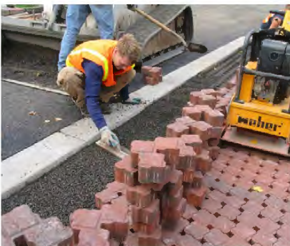
Pervious Pavement Construction
