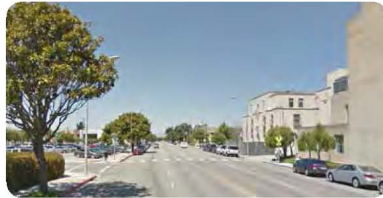
Existing Crossing on Alisal Street at Cayuga Street
