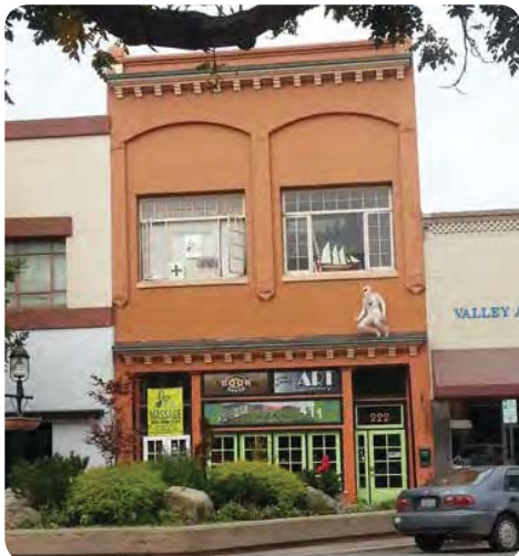
The Salinas411 building is a great example of a unique, active and intriguing storefront that attracts visitors and livens up the adjoining sidewalk space.
