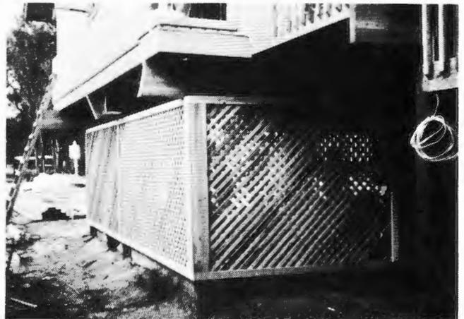
Figure 4.54. Breakaway Walls
