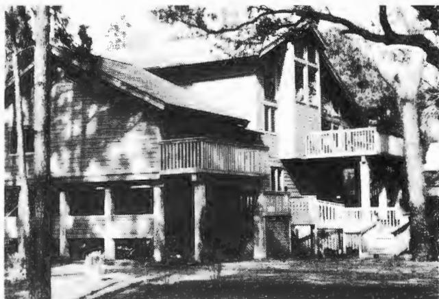
Figure 4.3. Elevation by Posts
