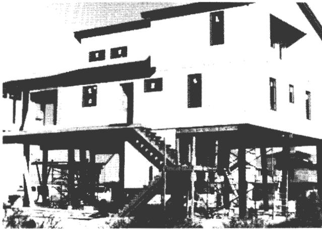
Figure 4.14. Pile Foundations
