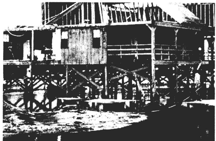
Figure 4.23. Diagonal Bracing
