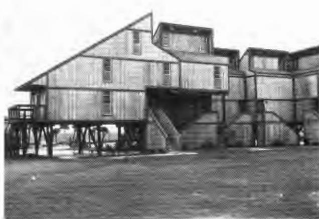
Figure 4.4. Elevation by Posts
