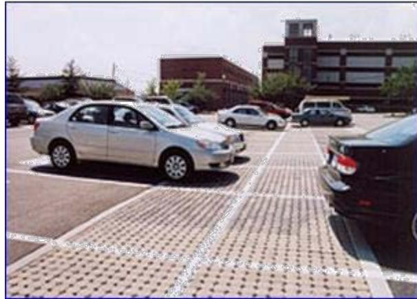
**Figure 3: Open Jointed Block Pavers**
