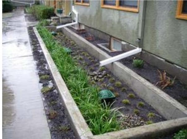
**Figure 7: Stormwater Planter (Source: Portland BES)**
