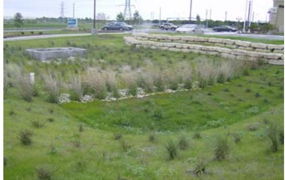
Figure 6: Biofiltration Basin (Source: Austin WPD)
