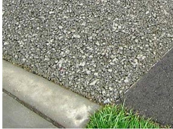
**Figure 4: Example of Porous Concrete (Source: LA LID Manual)**
