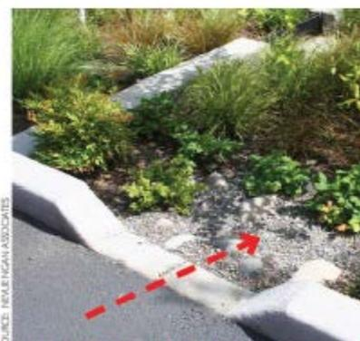
Figure 4-2: This standard curb cut at parking lot rain garden has 45 degree chamfered sides.
