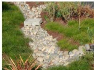
Figure 4-1: Cobbles in this stormwater treatment measure in San José help prevent erosion.
