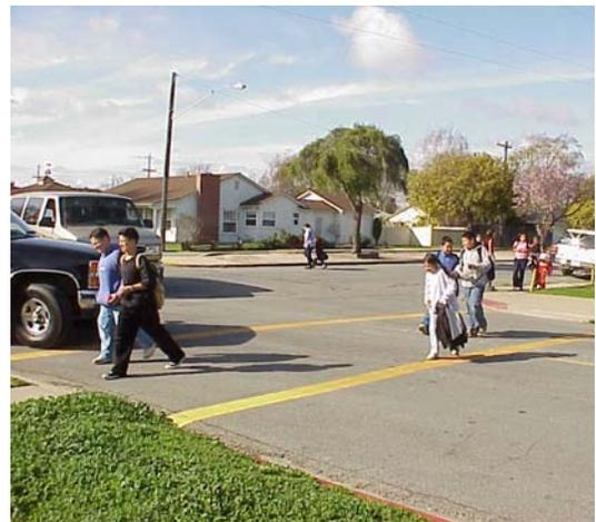
Installation of marked crosswalks at uncontrolled pedestrian crossing locations should not be regarded as a cure for pedestrian safety problems. However, marked crosswalks should also not be considered as a negative measure that will increase pedestrian accidents in all cases. Marked crosswalks are appropriate at some locations to help channel pedestrians to preferred crossing locations, but in many cases should be accompanied by other improvements.<sup>21</sup>
