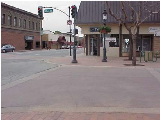
Curb returns are the curved section of curb when one street transitions to another (typically at an intersection). Alleys, lanes and streets in healthy neighborhoods should be designed for low turning speeds (6-10 mph).<sup>36</sup>
