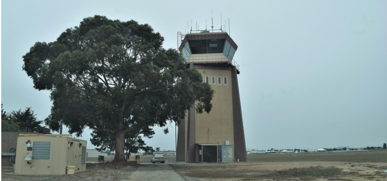
Figure 1.18 – SNS Airport Traffic Control Tower
