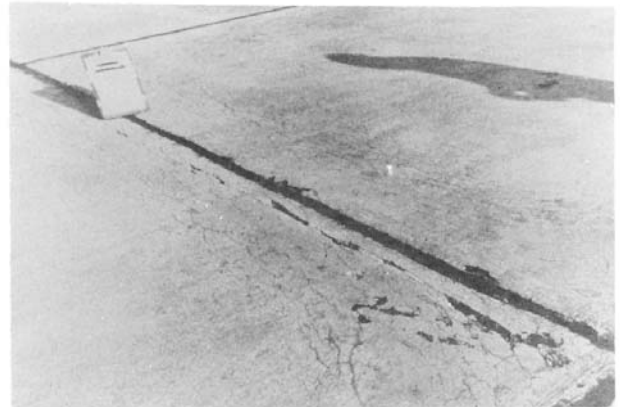
FIG. X2.22 High-Severity "D" Cracking
