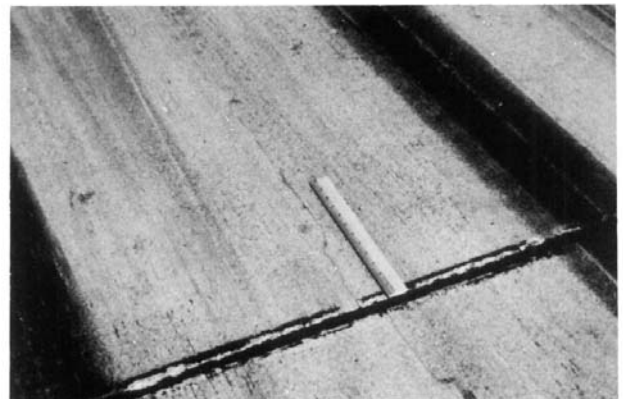
FIG. X2.58 Shrinkage Crack
