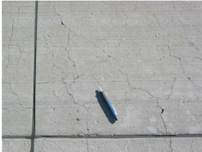
FIG. X2.75 Medium-Severity ASR
