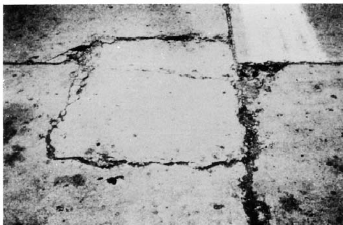
FIG. X2.37 High-Severity Patch
