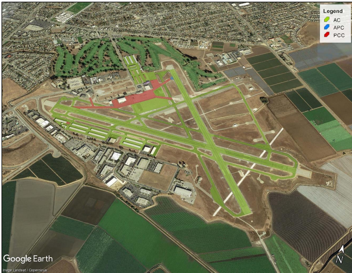
Figure 2.2.a Aerial Imagery with Pavement Surface Type
