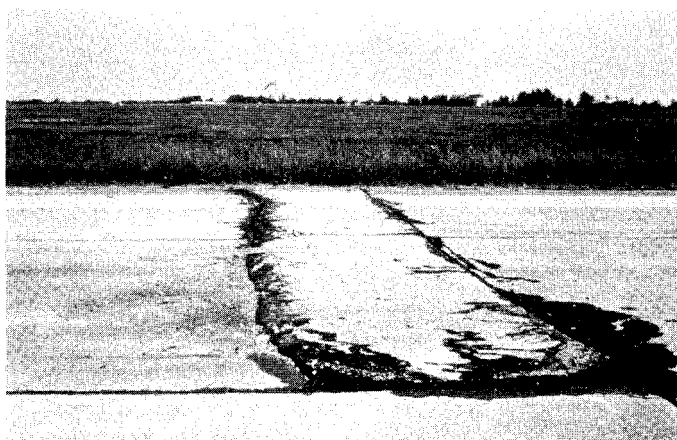
FIG. X2.2 Medium-Severity Blowup
