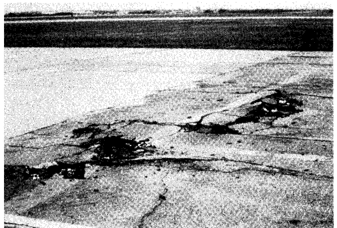
FIG. X1.72 High-Severity Shoving
