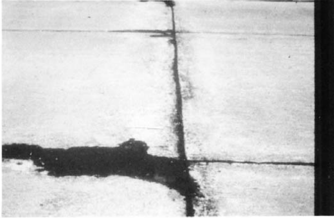
FIG. X2.45 Medium-Severity Scaling
