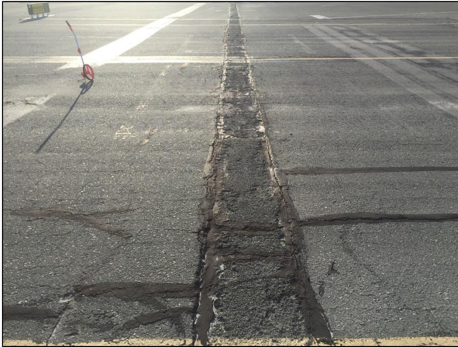
Taxiway D, Section 30 – Patch
