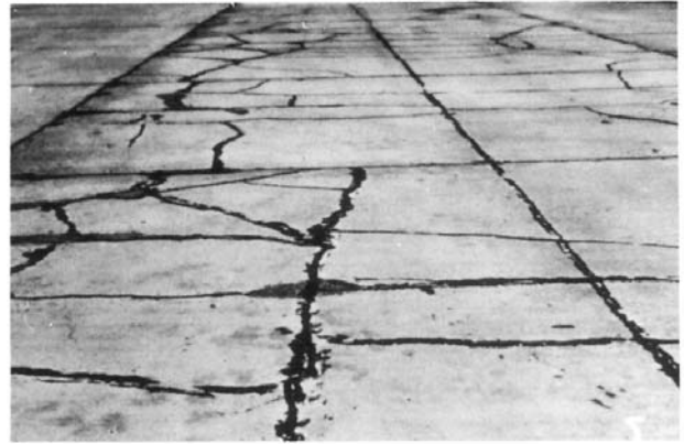
FIG. X2.57 Shattered Slab
