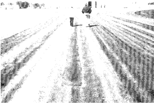
FIG. X1.48 Low-Severity Patch
