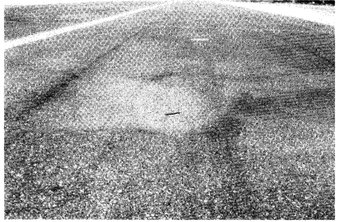
FIG. X1.26 Medium-Severity Depression
