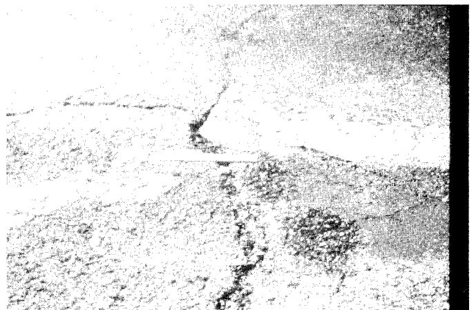
FIG. X1.42 High-Severity Longitudinal Crack
