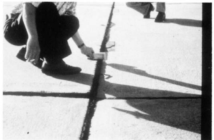
FIG. X2.52 High-Severity Settlement
