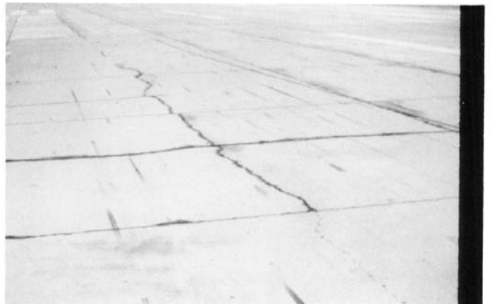
FIG. X2.53 Low-Severity Intersecting Cracks
