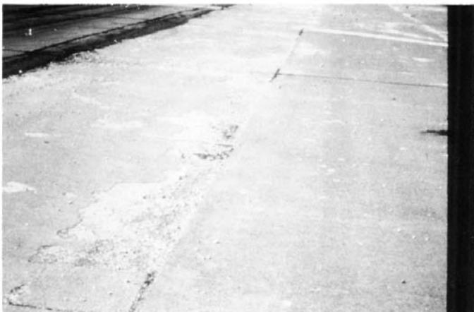
FIG. X2.46 High-Severity Scaling
