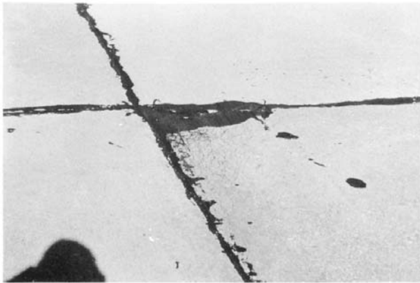
FIG. X2.19 Low-Severity "D" Cracking Approaching Medium Severity
