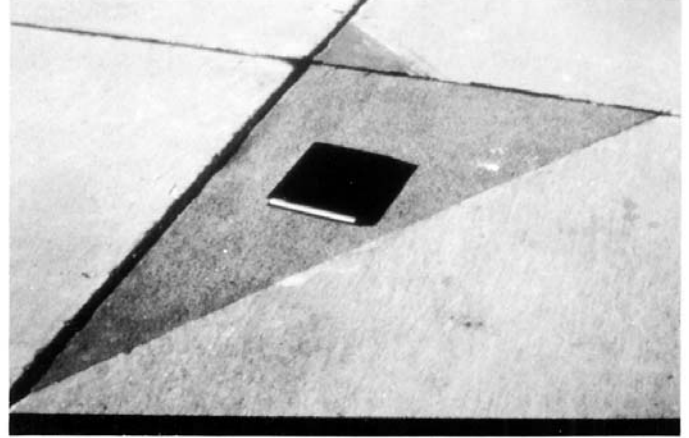
FIG. X2.33 Low-Severity Patch
