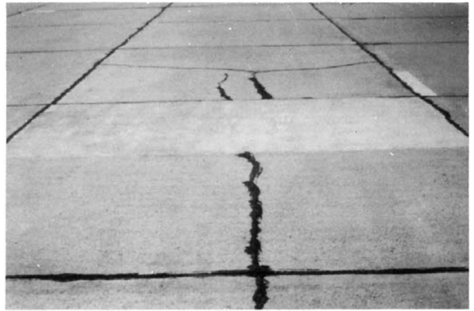
FIG. X2.34 Low-Severity Patch
