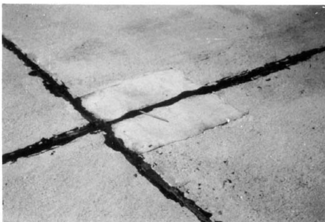
FIG. X2.28 Low-Severity Small Patch
