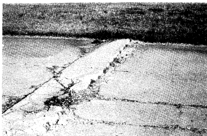
FIG. X2.3 High-Severity Blowup
