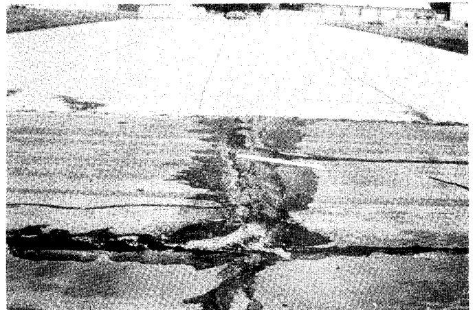
FIG. X1.78 High-Severity Swell
