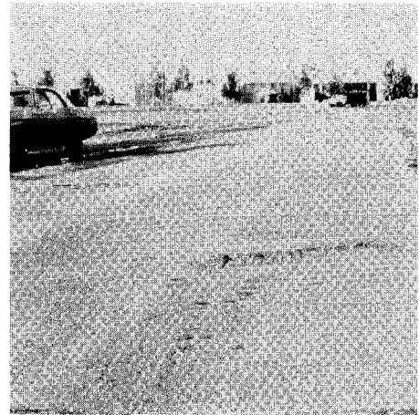
FIG. X1.77 High-Severity Swell
