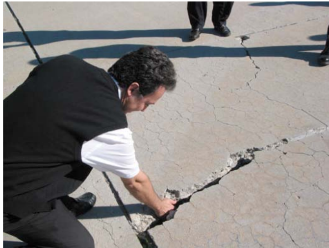
FIG. X2.76 High-Severity ASR
