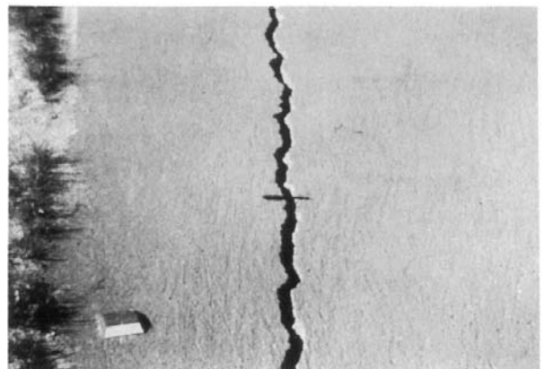
FIG. X2.17 High-Severity Crack
