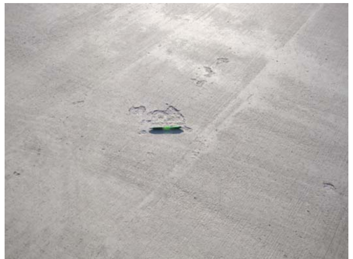
FIG. X2.44 Low-Severity Scaling
