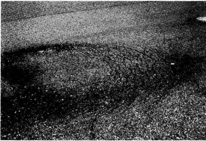
FIG. X1.73 Slippage Cracking
