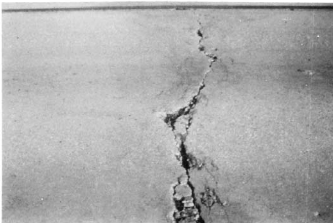
FIG. X2.15 High-Severity Crack
