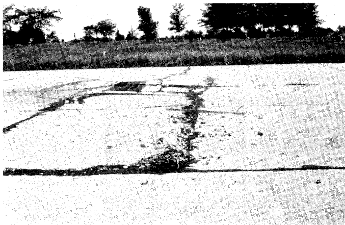
FIG. X2.1 Low-Severity Blowup
