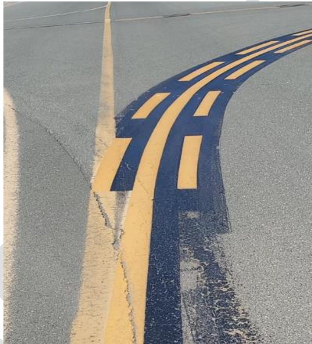
Figure 5.16 - Enhanced Centerline (Typical)
